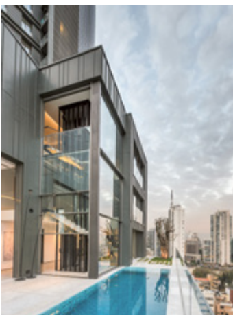
Project in Lebanon
